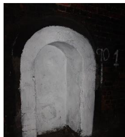
2A Refuge. Somewhere to avoid being crushed by a train
