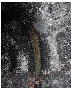
3The tunnel was mostly dry but not completely
