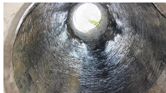
1One of the service tunnels now in someone's garden!
